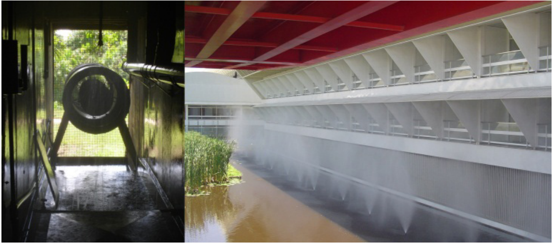
Figure 13. A misting system inside and outside the galleries in Salvador and Rio de Janeiro Sarah Hospital, respectively. Fonte: Marieli Azoia Lukiantchuki.
