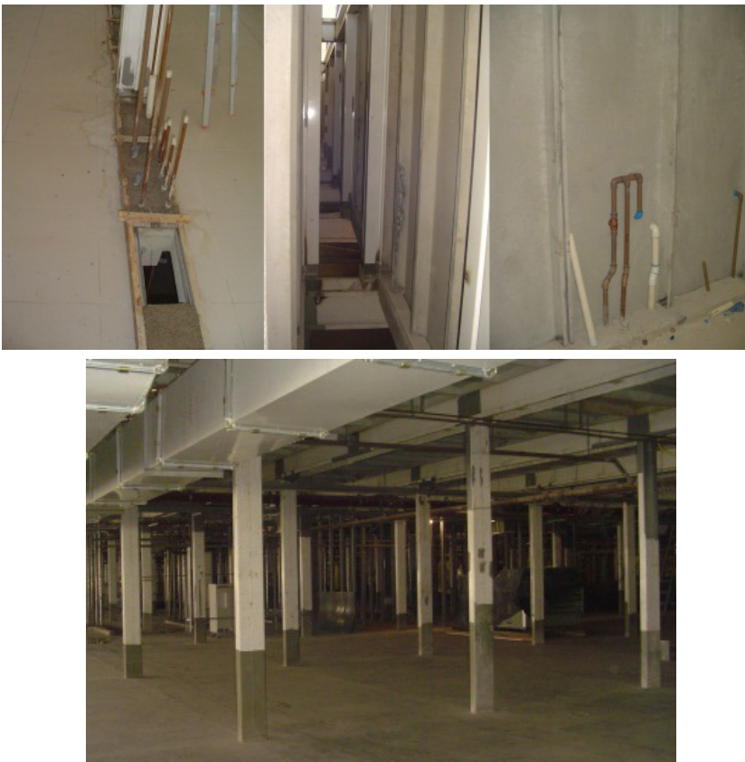
Figures 8 and 9. Precast ferrocement walls, double ferrocement panels and underground galleries of the Sarah Hospital of Rio de Janeiro. Source: Marieli Azoia Lukiantchuki.
