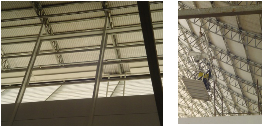
Figures 10 and 11. Walkways in great roof in sheds and equipment to facilitate the cleaning service located in the roof of the Sarah Hospital of Rio de Janeiro. Source: Marieli Azoia Lukiantchuki.
