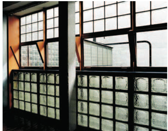
Figure 4: Maison de Verre. Tilting window frame in the laundry. Source: Mark Lyon, authorized photographer Maison de Verre - www.marklyon.fr - www.marklyon.fr .
