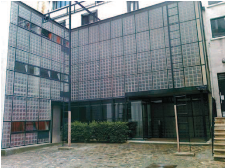
Figure 1: Maison de Verre. Front view: glass block panels that give the building the name by which it is known - entry access to the house-clinic. On the right side of the image, you can see the stairs that lead to the third floor: an apartment independent of the Maison de Verre. Source: Author, 2011.
