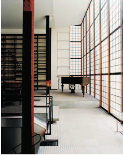
Figure 5: Maison de Verre. Grand salon - in the background, tilting vertical frame which regulates the ventilation of the room, Source: Mark Lyon, authorized photographer Maison de Verre - www.marklyon.fr
