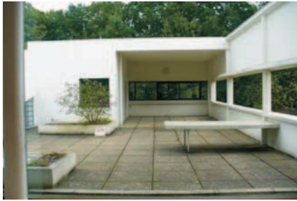
Figure 18:Villa Savoye. External terrace. Source: Author, 2011.
