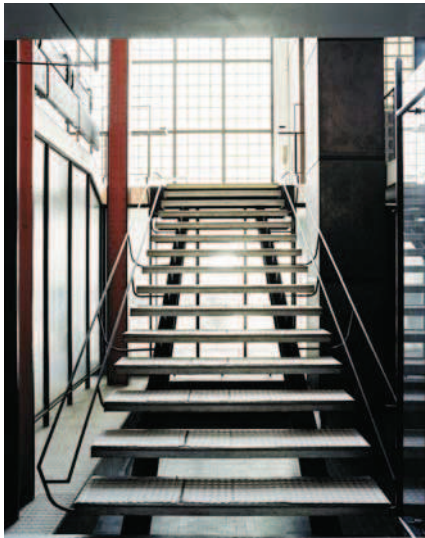
Figure 7: Main staircase that gives access to the grand salon of the house. Source: Mark Lyon, authorized photographer Maison de Verre - www.marklyon.fr
