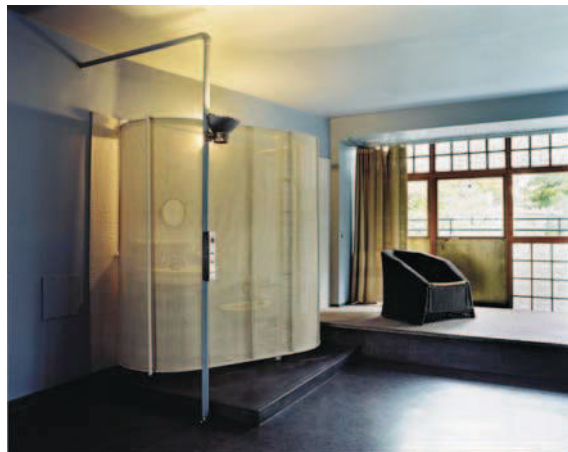
Figure 9: Maison de Verre. Sink and bidet, hidden by metallic screen panel. Source: Mark Lyon, authorized photographer Maison de Verre - www.marklyon.fr
