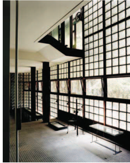
Figure 6: Waiting room of the clinic, at the back of the house. Glass block panels combined with tilting frames. Source: Mark Lyon, authorized photographer Maison de Verre - www.marklyon.fr
