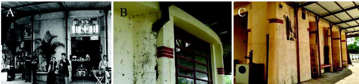
Figure 7: Original pluvial conductors and the loss of the element on the façade. Source: A (CONDEPHAAT, 1986), B (SECRETARIA DA CULTURA, 2014) and C (Authors' collection, 2016).
