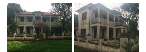
pedestals and access staircase, masonry in massive bricks, with panels covered with mortar.
