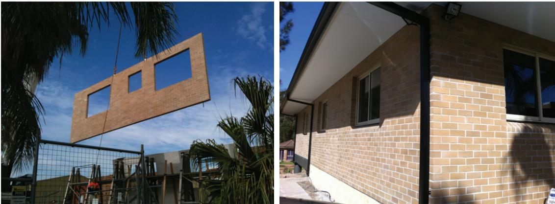
Figure 5. Prefabricated housing system.
