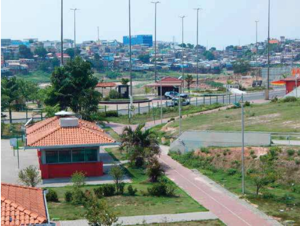
Linear Park in Manaus, part of the urban requalification program called Programa Prosamim . Manaus, AM, Brasil. Source/picture: Eugenio Fernandes Queiroga, 2015.
