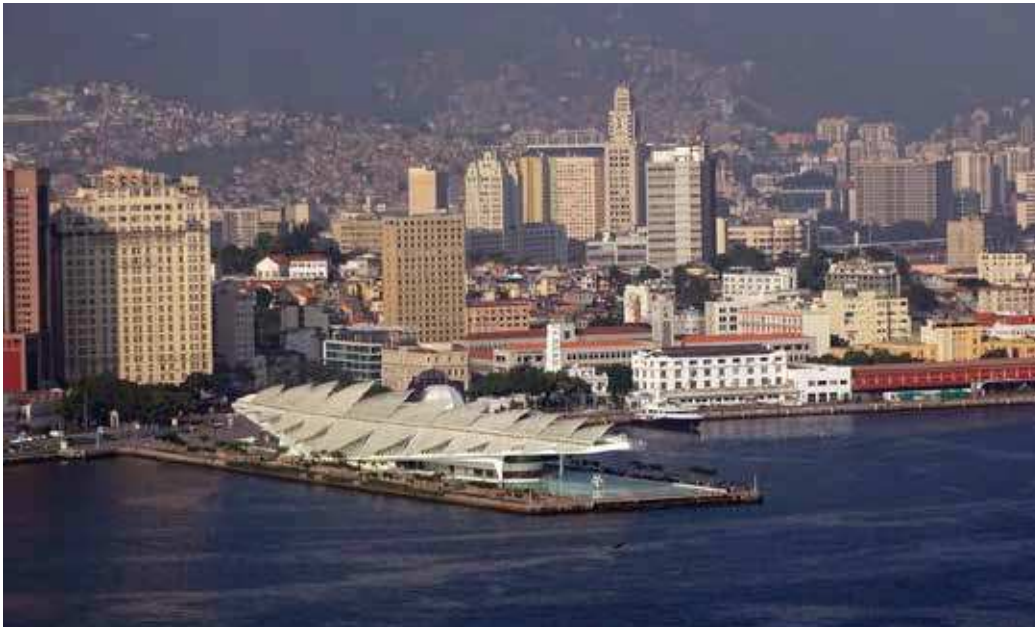
View of Porto Maravilha, Museu do Amanhã in the front. Source/picture: Silvio Soares Macedo, 2016.
