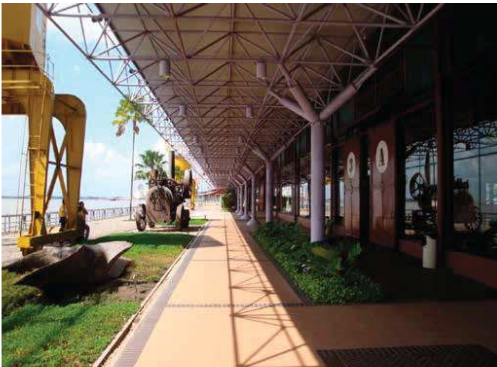
Estação das Docas , Belém do Pará, a small fragment of the city's port waterfront is open to the population, by means of a high quality design and landscaping project, although its use is restricted mostly to tourists and high-income population. Source/Picture: Leonardo Coelho, 2014.
