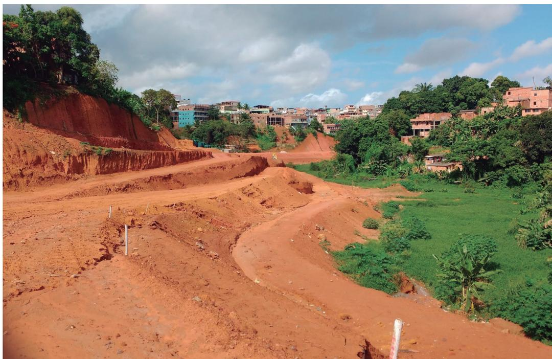
Figure 1: Construction of the Mário Sérgio Avenue on the Mocambo River PPA, with floodplain on the right side.
