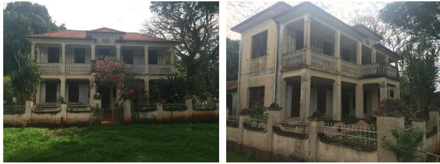
pedestals and access staircase, masonry in massive bricks, with panels covered with mortar.
