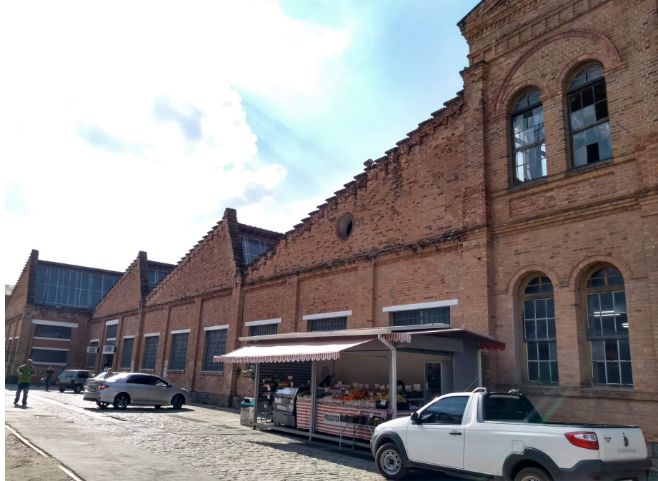
Figure 6 – External view of the Northern Section. Note the different openings that made up the lighting and ventilation system: shed, windows and oculus. Fonte: Source: Author's personal collection, 2018.
