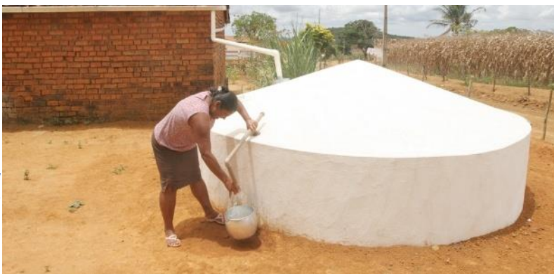
Figure 2: Cement slab cisterns in the Brazilian semi-arid region. It is an appropriate use of a technoscientific cement solution to the local reality. Source: Jornal GGN, 2012. https://jornalggn.com.br/politicas-sociais/comunidades-criticam-as-cisternas-de-plastico/
