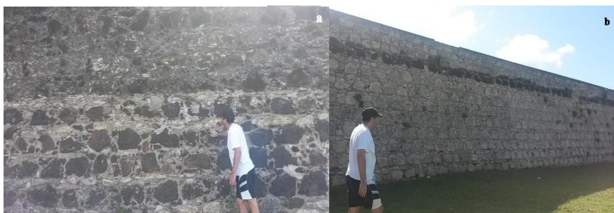
Figure 6: Elements of ex situ geodiversity present in the Fortress of Cabedelo. (a) Wall composed primarily of ferruginous sandstones; (b) Wall with limestone blocks and an upper line with Ferruginous sandstones. Photos: Ingrydy Pereira.
