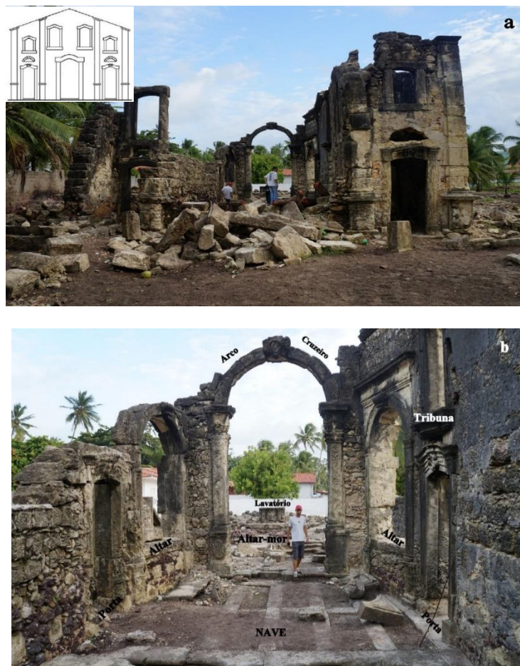
Figura 4: Ruins of Almagre. a) View of the front facade and, in detail, model of the complete facade. Note that the tower wedges are in danger of collapse; b) Detail of some internal components of the church. Photos: the author.
