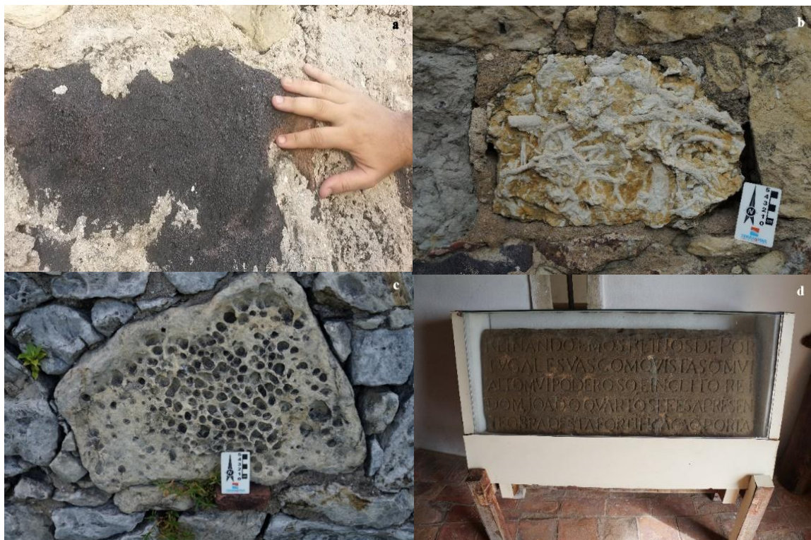
Figura 7: Detail of the rocks from the walls of Fortaleza de Cabedelo. (a) Ferruginous sandstone; b) Limestone of the Gramame Formation with ichnofossils; (c) Honeycomb lapies; d) Carved Ferruginous sandstone. Photos: the author.
